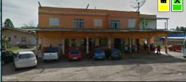
HOTEL E RESTAURANTE - SENTIDO SANTA MARIA km 156+700 S: 29°43'56.81" O: 52°56'49.80"
