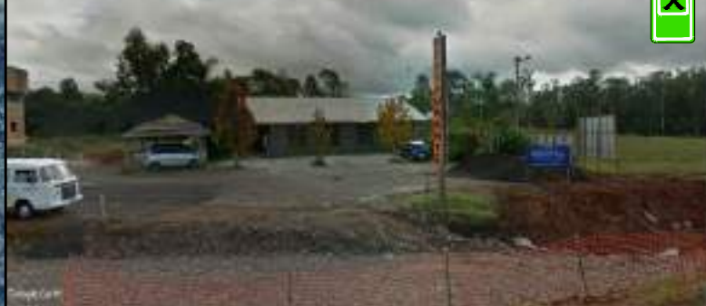
RESTAURANTE - SENTIDO SANTA MARIA km 157+430 S: 29°44'10.43" O: 52°57'15.21"
